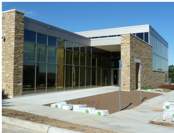
Shown on July 15, construction is nearly complete on the new Helmerich Center for American Research. The Grand Opening Celebration is planned for September 6 and 7. (Photo by Dana Simon)
